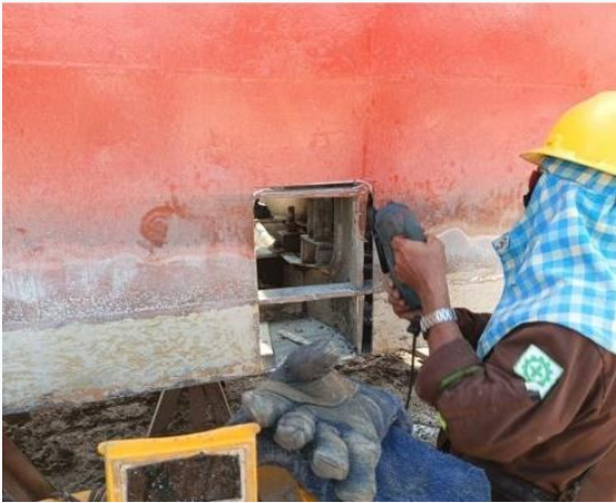
BEFORE / OPEN CUT-OUT
